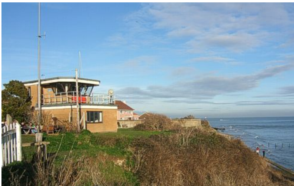
The site of Fort Ground as it is today looking north-east towards Forelands.
